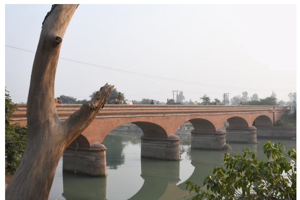
Figure 20: View of the Sankara bridge Source : As per primary survey done on site
