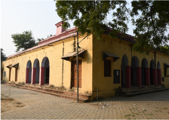
Figure 17: External facade of the Shree Krishna Inter-College Source : As per primary survey done on site
