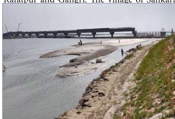
Figure 5: Sankra Ganga bridge and ghat
